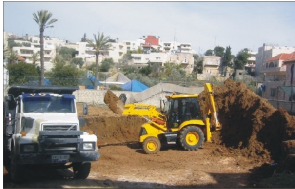
Day one of excavation
